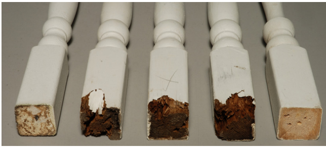
Figure 16–16. Cedar heartwood porch styles removed from a railing after 25 years of service. All the styles where end grain was primed before assembly were in perfect condition (left). All the styles without primed end grain on the bottom (center 3) were rotten. The top of a style without primed end grain is shown on right—it was protected from water and so performed perfectly.
