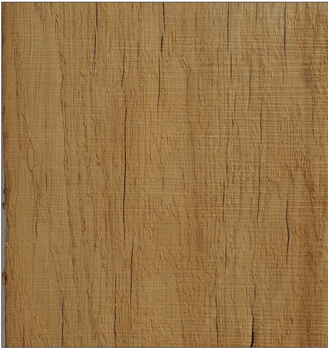
Figure 13-8. Surface checking on white oak 5/4 lumber.
